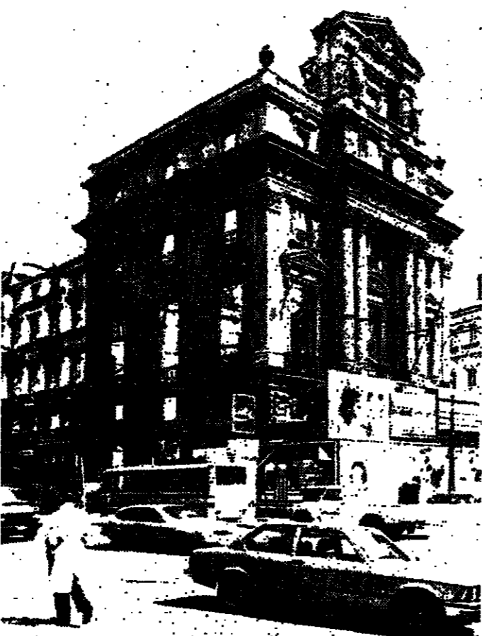
While retaining the classical exterior of this Ministry building in the Place de Brouckere in Brussels, the interior was totally rebuilt at a cost equivalent to BF31,500 (£366) per square metre. The 13,500 sq metres of space in the building includes offices, shops, residential and commercial areas
